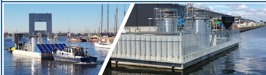
Treatment plants on a floating pontoon
