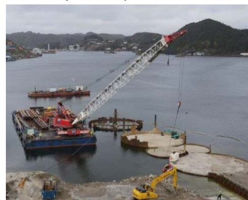
Foto: Fundamentering AS
