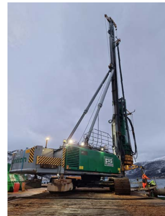
Foto: Fundamentering AS
