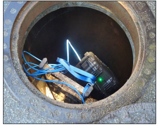
Figure 1. Installation of flowmeters inside the upstream and downstream manholes of the studied area
