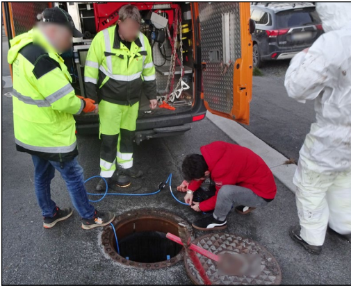
Figure 1. Installation of flowmeters inside the upstream and downstream manholes of the studied area
