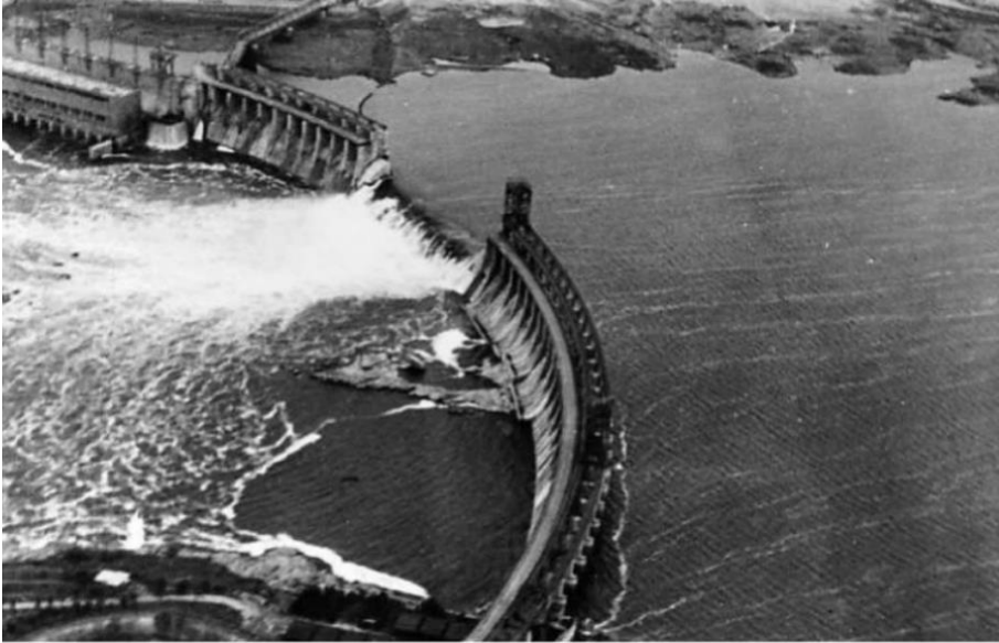
The dam on the Dnieper River near the city of Zaporizhzhia after reportedly being blown up by Soviet special forces in 1941 in an attempt to delay the offence of German troops
