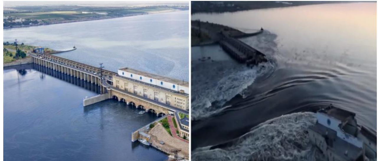
Kakhovka Dam on the Dnieper river, damaged in June 2023
