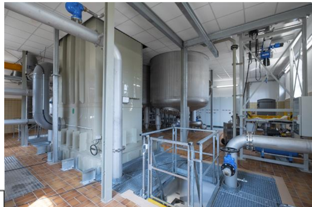
Energy intensive reverse osmosis facility to eliminate PFAS at the Rastatt test site to make drinking water potable
