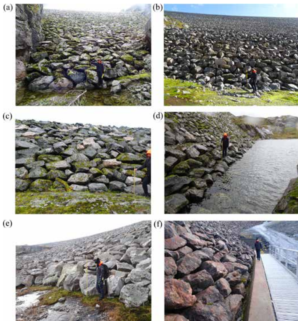
Figure 7. Depiction of existing conditions of placed riprap toe sections. Category 1 at dams (a) Fjellhaugvatn dam (b) Oddatjørn dam and (c) Skjerjevatnet main dam. Category 2 at (d) Skjerjevatnet main dam. Category 4 at (e) Storvass dam. Category 5 at (f) Akersvass dam.
