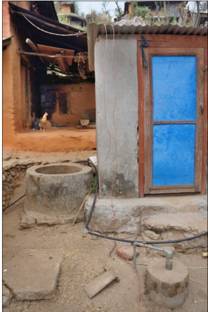
Toilet connected to biogas reactor
