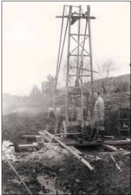
Figure 2. Cable-tool-percussion drilling.
