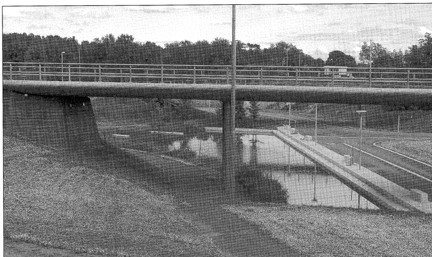
Dam i veianlegg
