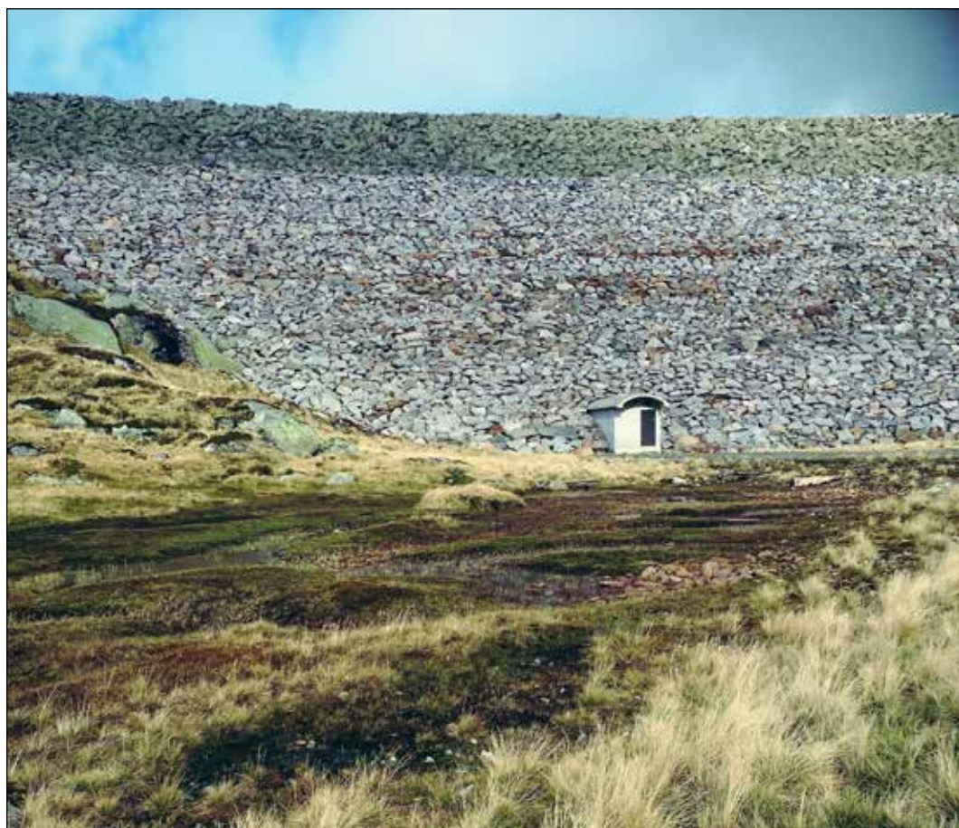
Dam at Roskreppfjord
